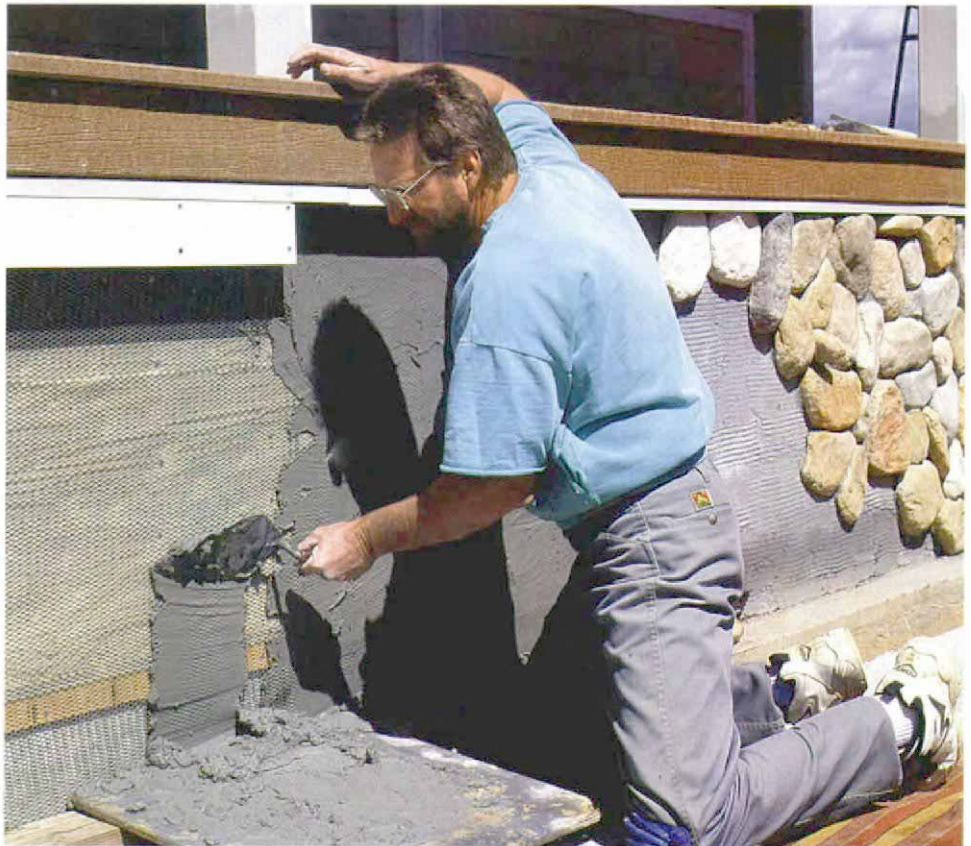
A textured finish provides better grip. A notched trowel creates a furrowed surface that is better for bonding the manufactured stone to the wall.
