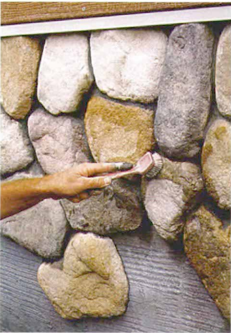
A gentle hand with a soft brush. The color on the surface of manufactured stone can be damaged with abrasives or acid, so excess mortar must be brushed off lightly with a soft brush.
